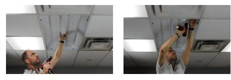
**STEP NINE:** Re-install the lens door frame.
